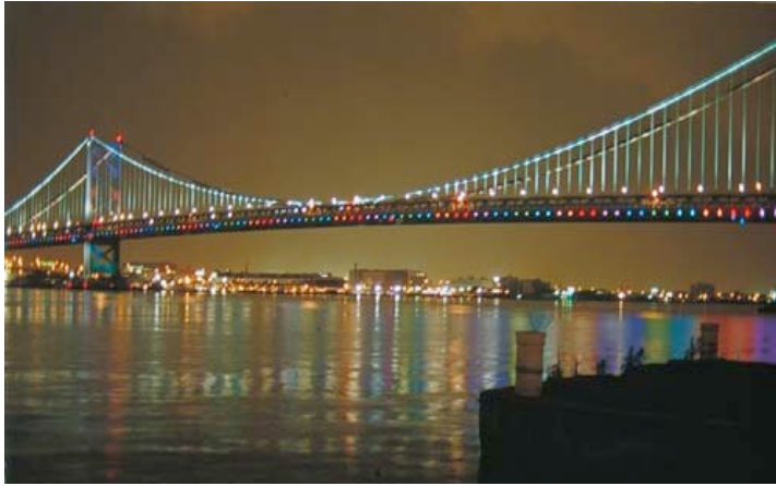
Installation Benjamin Franklin Bridge, PA, USA (Color Kinetics Inc.)
