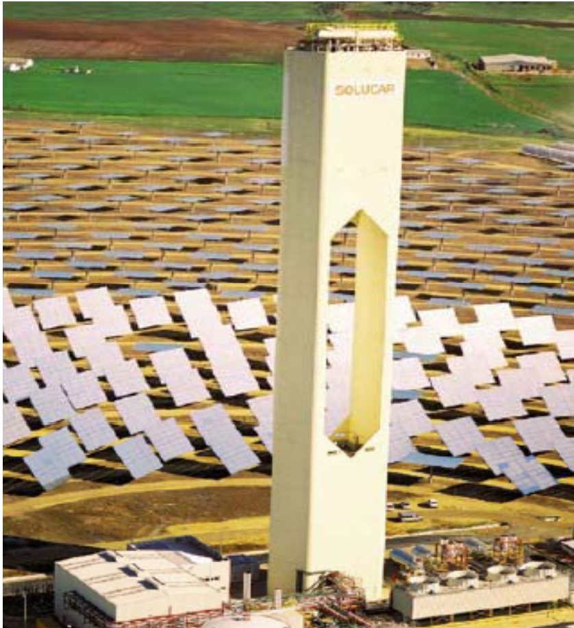
Figure 1: Above, power tower pilot project, pioneered in the U.S. (Barstow, CA) and (left) commercial unit under development by Abengoa called PS10, an 11 MW plant in Sevilla Spain (photo credit: Abengoa Solar). Bottom left, Stirling Dish/Engine, Center SEGS trough plants, Right, Compact Linear Fresnel Reflector.
