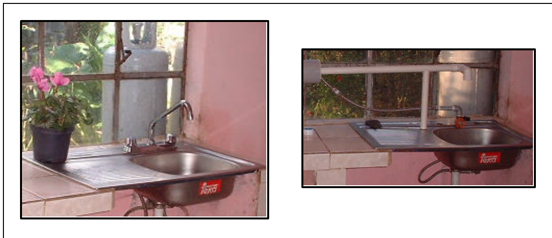
Figure 34 Picture of Installation Site Before and After
