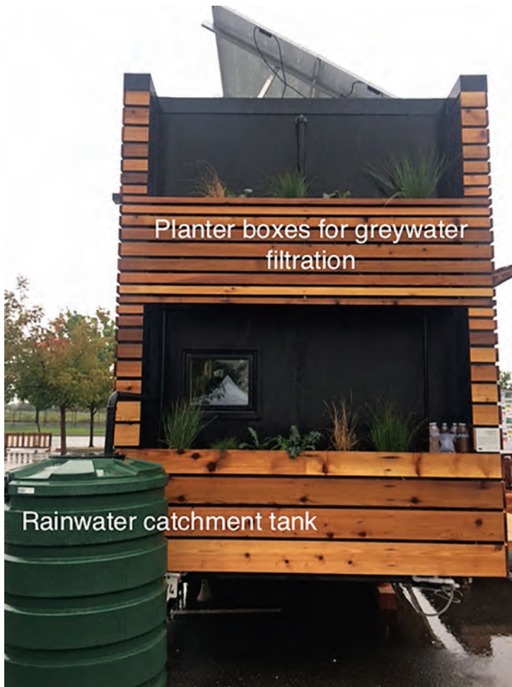
FIGURE 4. Water filtration and catchment system.
