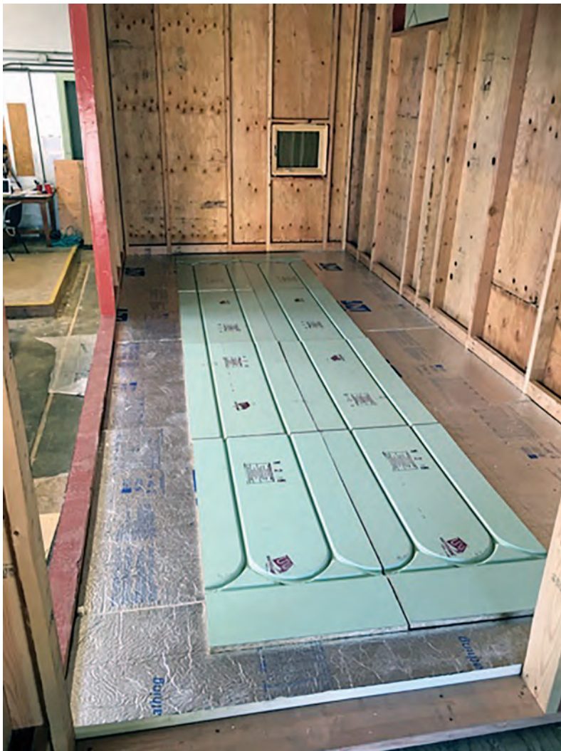
FIGURE 3. THIMBY Warmboard Radiant Floor Layout.
