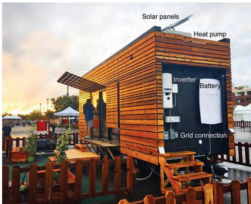
FIGURE 1. THIMBY Energy System Components.
